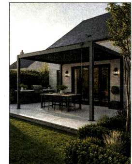
Image of demountable/ Temporary structure
